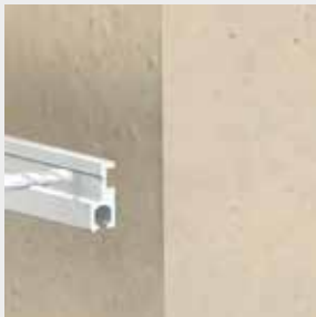
1. Drill hole in track
