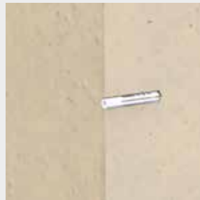
2. Insert suitable dowel
